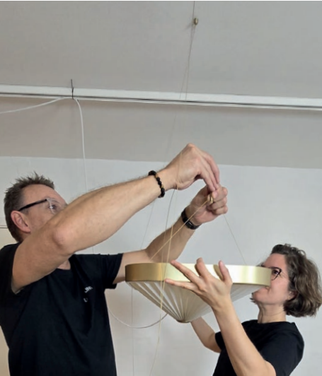
31. Here you will need one person to hold the lamp in position, while the other person attaches the thin suspension wires and do the adjustments.
